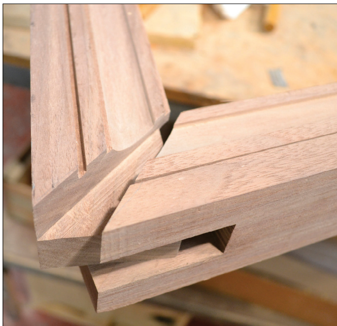
● The rain sill frame's top corners go together with a classic bridled miter.
